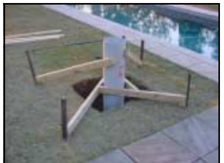
Figure 3: Formwork
